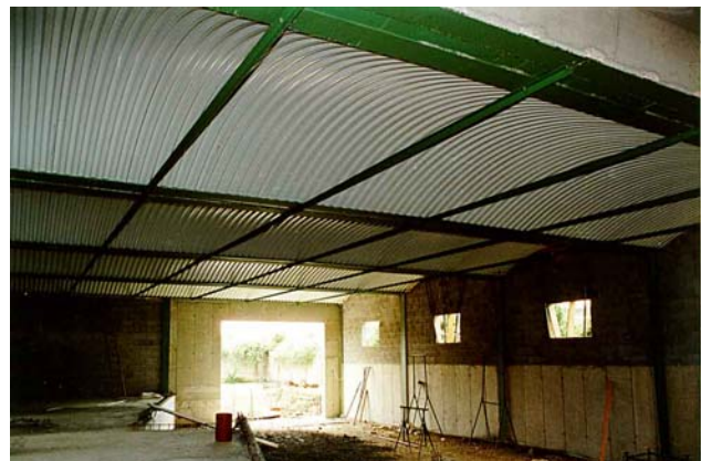
Soffit of finished floor right after concreting
