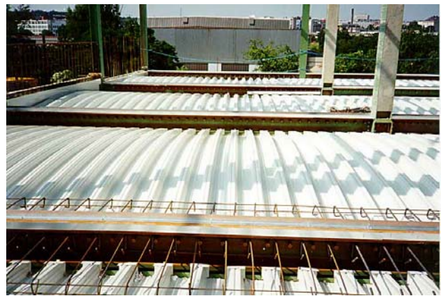
Trapezoidal arched sheets before concreting
